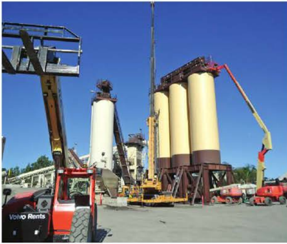
Above: Installation of the new Astec Storage Silos and scale at BoDean's Santa Rosa facility. These 300-ton capacity Astec silos and the new scale represent just some of the many technological additions and modifications being added to the BoDean Company asphalt plant located in Santa Rosa Calif.
