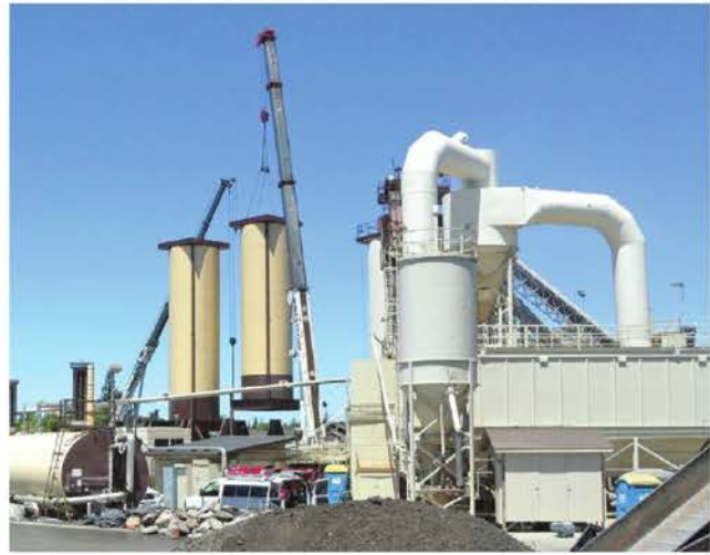
Above: Installation of the new Astec Storage Silos and scale at BoDean's Santa Rosa facility. These 300-ton capacity Astec silos and the new scale represent just some of the many technological additions and modifications being added to the BoDean Company asphalt plant located in Santa Rosa Calif.
