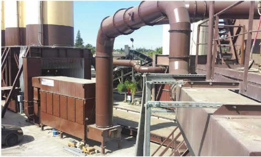
Above: BoDean Company recently installed Blue Smoke Collectors manufactured and installed by Butler Justice, Inc. on the new and existing silos and on the existing plant. Blue Smoke Control is a patented product of Butler Justice, Inc. and is necessary to filter and help eliminate asphalt odors and fumes from entering the atmosphere.
